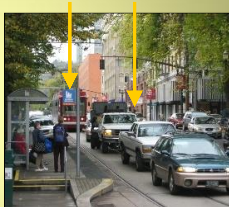
Fifth Street after reopening, Portland, OR
