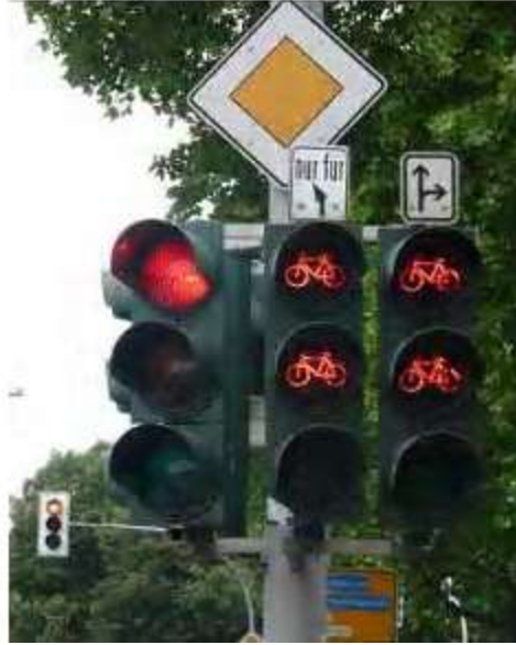
• Typical traffic signal in Muenster, where cyclists usually get an advance green light ahead of motorists
